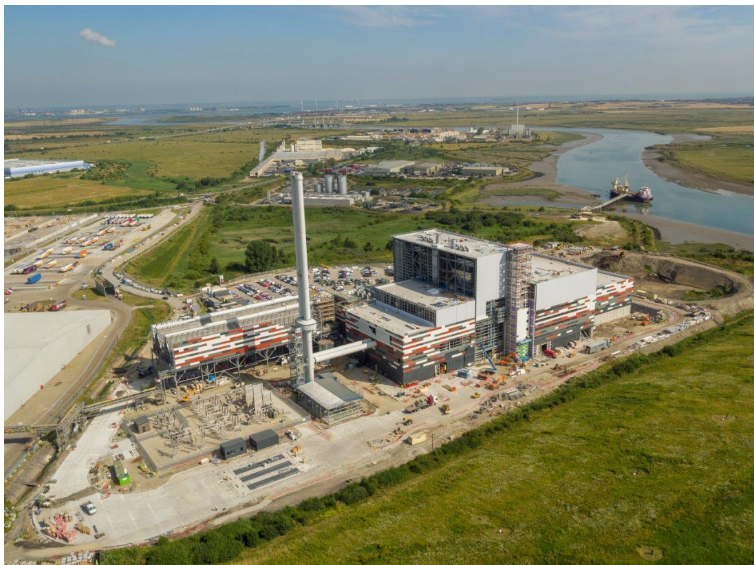
Figure 6.1 – K3 construction progress at July 2019.
